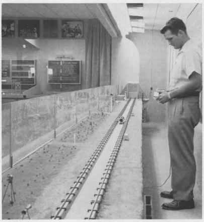
ROCKET SLED TESTS performed with a model operated by James R. Winchell, of the Test Laboratory Department, have numbered in the hundreds. Complete with sound effects, the tests thrill onlookers with both colorful and spectacular demonstration of speed.
